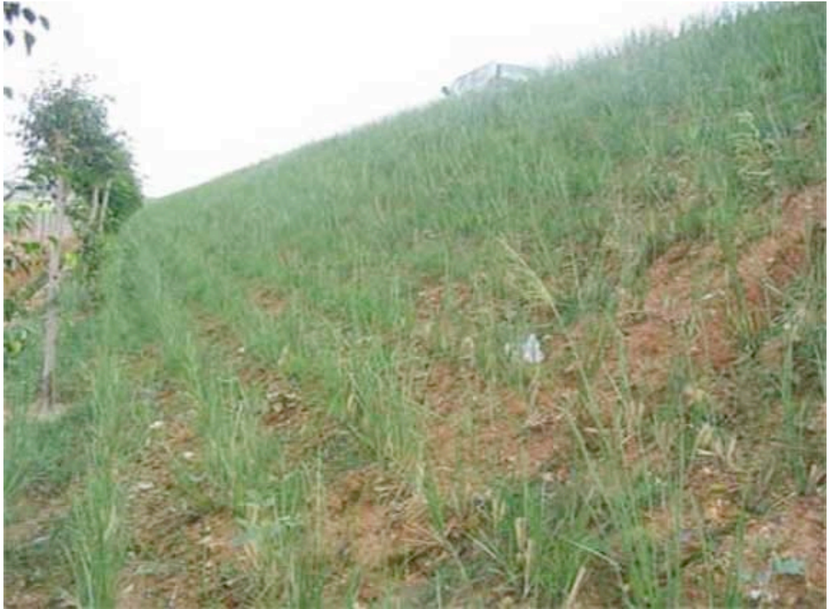
Vetiver and other grasses, such as bahia grass, began to cover the slopes 2~4 months after planting.
